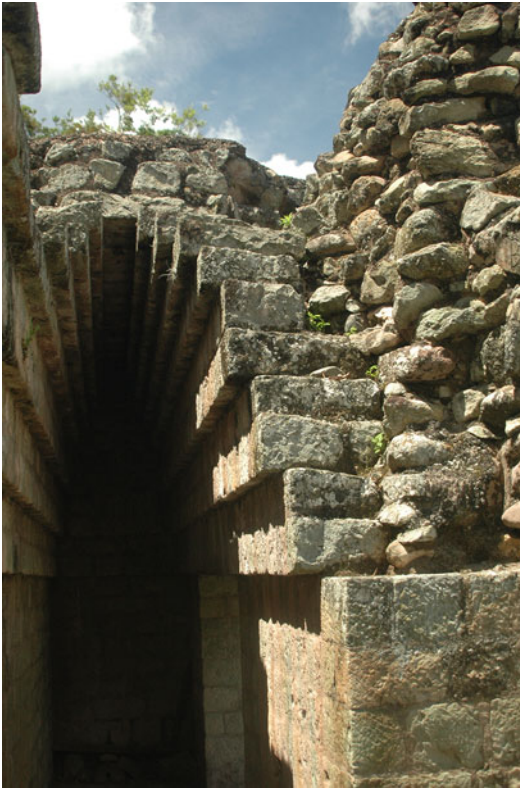
Architecture of the Maya: Public Architecture, Fig. 1 View of poorly preserved masonry showing interior masonry fill and exterior finished stones in the ballcourt building of Copan, Honduras
