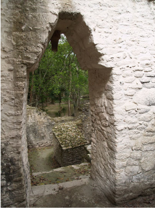
Architecture of the Maya: Public Architecture, Fig. 7 Doorway with corbel arch at Cahal Pech, Belize
