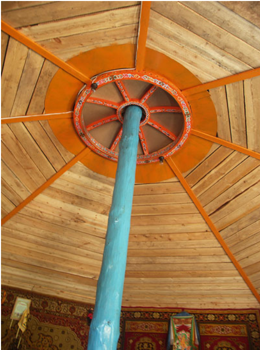
Architecture: Nomadic Architecture of Inner Asia, Fig. 49 Inside a wooden house resembling a ger. In this house even a roof wheel has been used. Mongolia, Terelj
