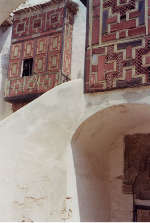
Architecture in Suakin, Fig. 8 Color view of rawashin as reerected in the Muhafaza courtyard in the 1930s, removed from deteriorating private houses on the island. These are late examples of simplified and inferior construction but indicate the contrasting colors typical of the decorative woodwork involved. These colors also are indicated in Fig. 2 (© SARS Greenlaw Archive GRE P147.03)
