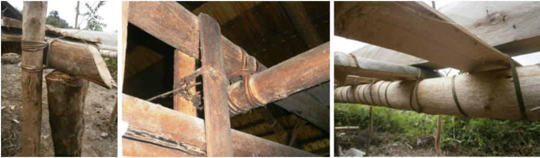
Architecture of the Moluccas, Fig. 5 Left: A structure formed of connected single poles; Middle: connected walls; Right: connected floor
