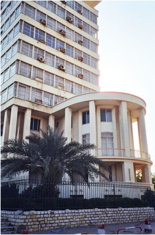
Architecture in French West Africa, Fig. 9 Dakar, Senegal. The governmental building administratif , the 1950s (Author’s photo)
