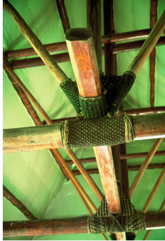
Architecture of Fiji, Fig. 40 Beautifully lashed joints of a roof structure on Bau island
