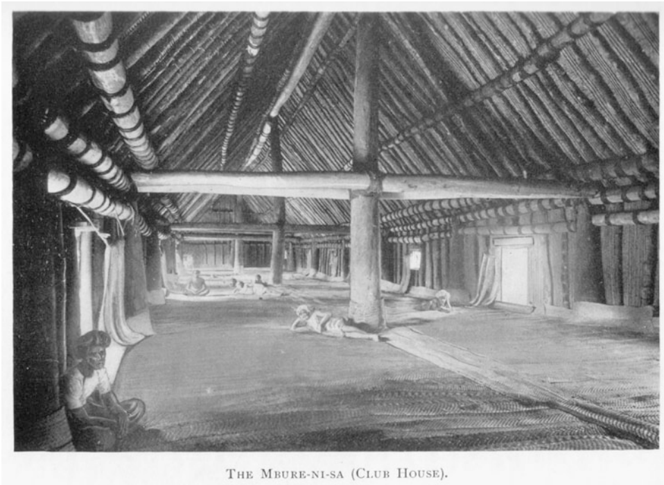
Architecture of Fiji, Fig. 20 Bure ni Sa on Bau island (Source: Thomson, 1908). This example is a very large and generous one. Bure ni Sa in the highlands for example seem to have been much smaller and had a rather confined
