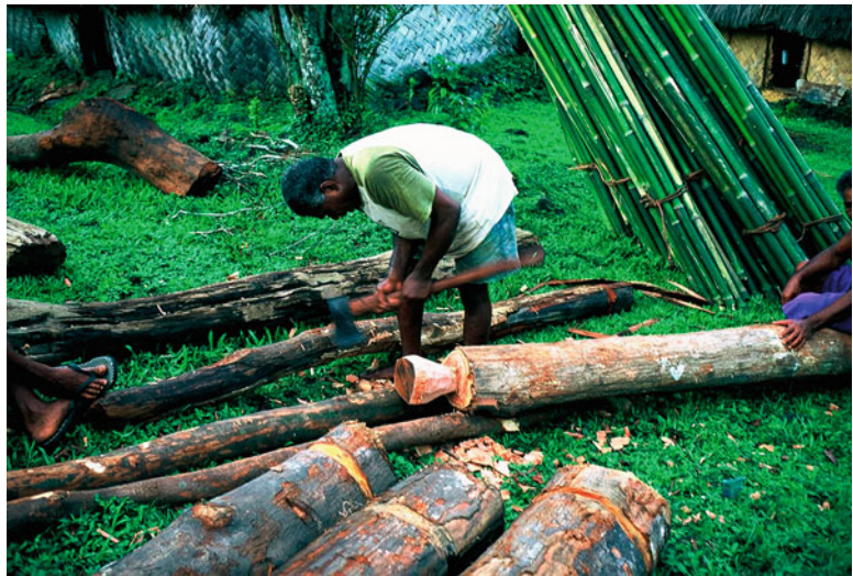
Architecture of Fiji, Fig. 32 Notching of the piles
