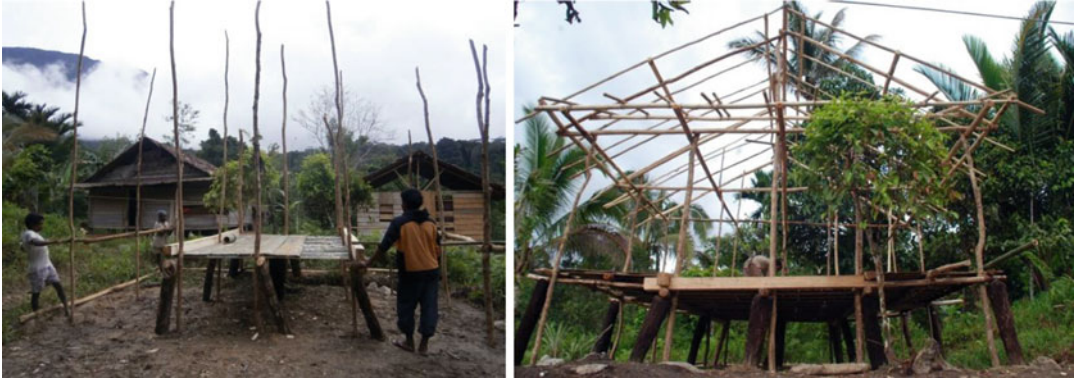
Architecture of the Moluccas, Fig. 3 Left: Installing the pillars; Right: pine wood in a diagonal position
