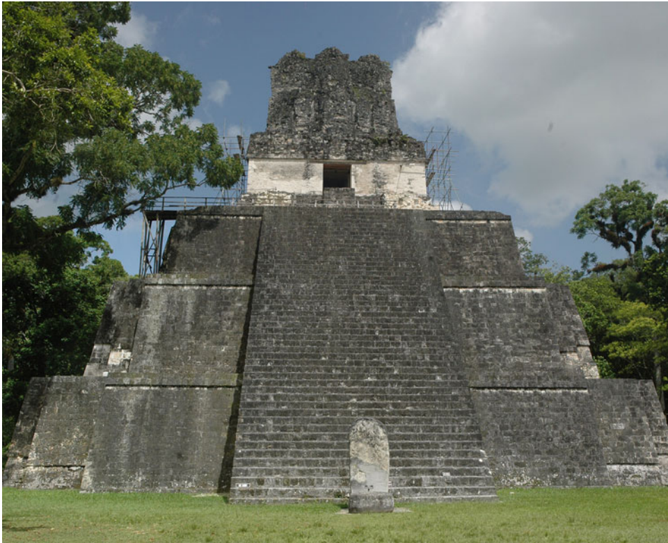
Architecture of the Maya: Public Architecture, Fig. 2 Temple II of Tikal, Guatemala. The three substructural sections of Temple II support its single-roomed superstructure with massive roof combs
