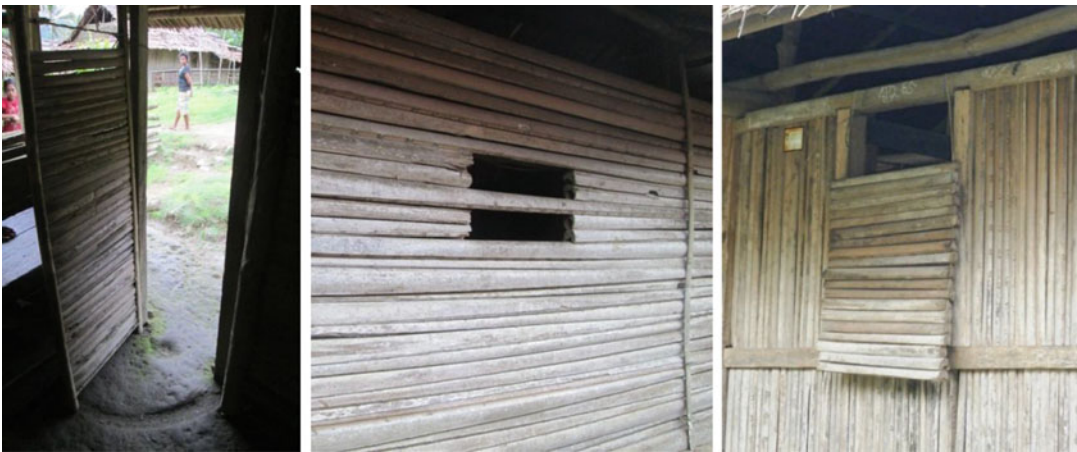
Architecture of the Moluccas, Fig. 6 Left: Door; Middle; window for the semipublic room; Right: window for the private room
