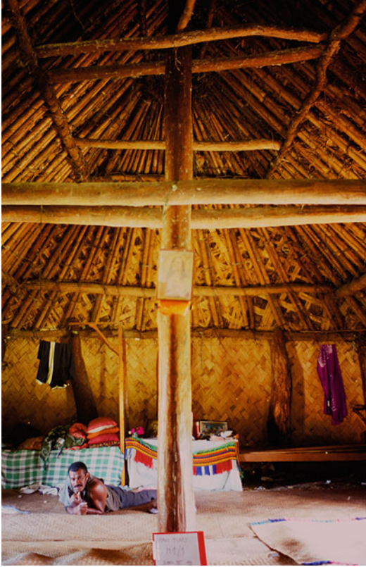
Architecture of Fiji, Fig. 11 Vernacular house with middle post in Navala village, Ba
