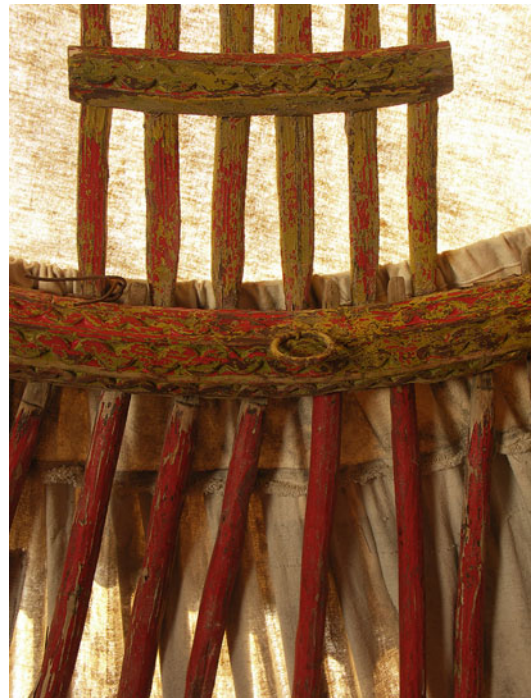
Architecture: Nomadic Architecture of Inner Asia, Fig. 36 Detail of a roof wheel of an Uzbek yurt (Source: Erich Lehner). The rim of such wheels is steamed and bent to a circular shape. The roof wheel of Mongolian gers is assembled from several pieces and not bent
