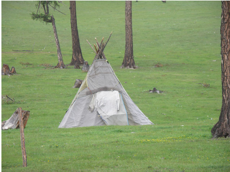
Architecture: Nomadic Architecture of Inner Asia, Fig. 2 Tent with load-bearing wooden inner structure, N-Mongolia
