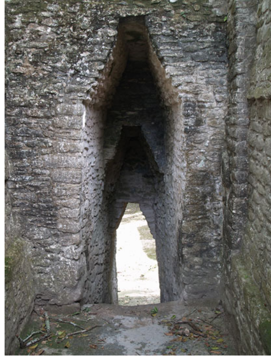
Architecture of the Maya: Public Architecture, Fig. 8 Corbel vaulted interior stairway at Cahal Pech, Belize
