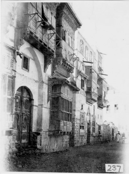
Architecture in Suakin, Fig. 2 Street scene of several houses, including Beit Sayd el-Safi (House 225) on the left, showing the variety of rawashin and other exterior decoration. Shish -work is best seen at center left. Note the added vertical bars on the ground-level rawashin and windows and the deteriorating walls at ground level (© SARS Greenlaw Archive GRE P034.01)
