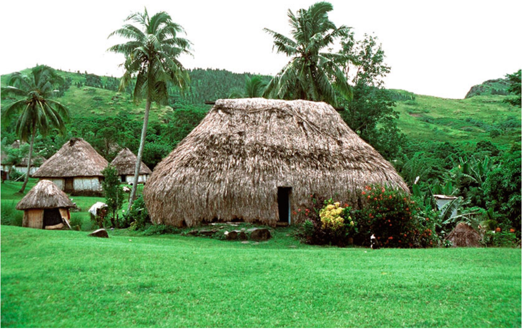
Architecture of Fiji, Fig. 8 Rectangular house showing many characteristics of the extinct Were Rausina building type. Navala village, Ba
