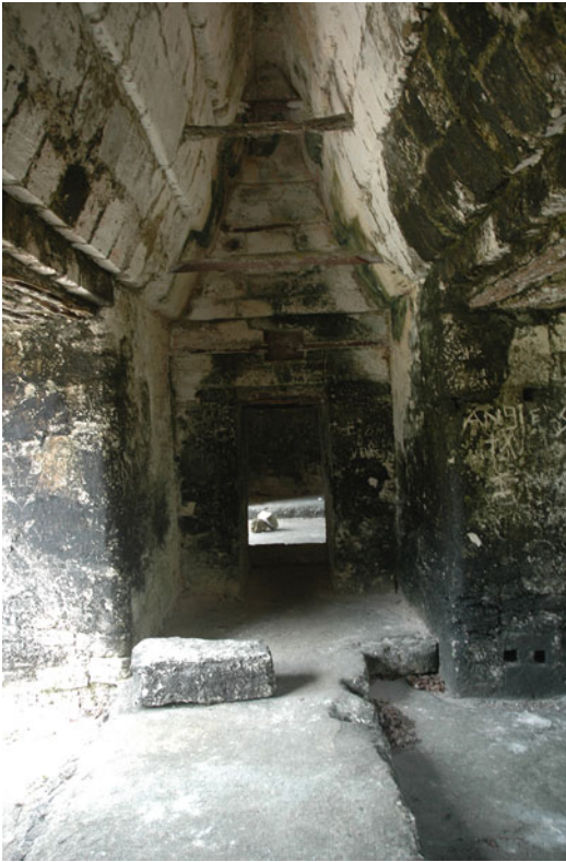
Architecture of the Maya: Public Architecture, Fig. 9 Corbel vault and room interior in the Plaza of the Seven Temples at Tikal, Guatemala, showing plastered surfaces, floor elevations, and vault beams
