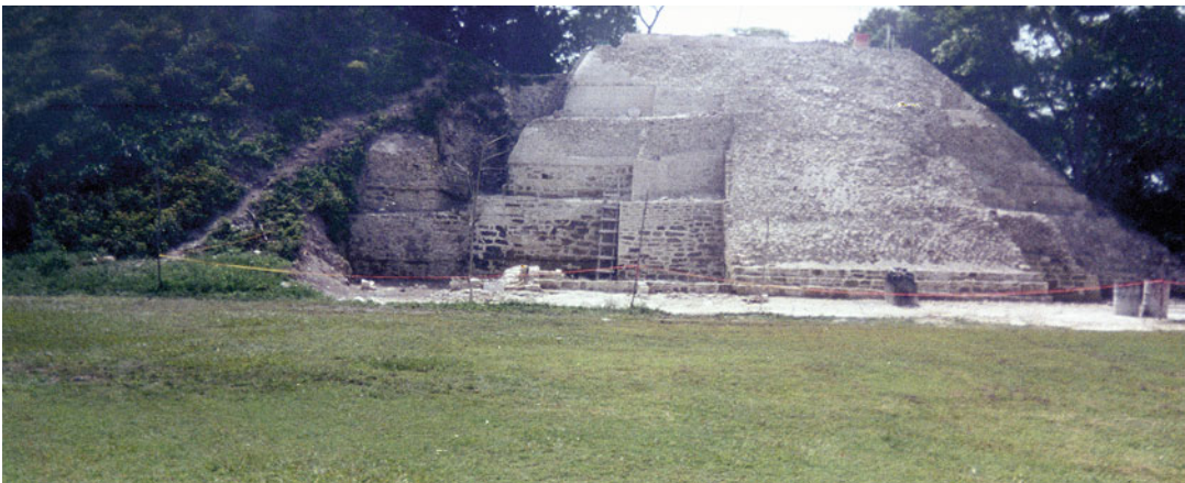
Architecture of the Maya, Fig. 2 Step pyramid being reconstructed at Xunantunich, Belize, in 2001. On the right side, the building facade is collapsed while on the left is a partially restored structure
