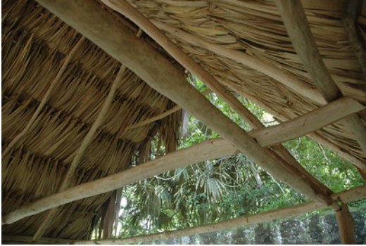
Architecture of the Maya: Domestic Architecture, Fig. 1 View up into a modern roof structure at the archaeological site of Tikal showing perishable materials, supporting wooden members, and covering palm thatch
